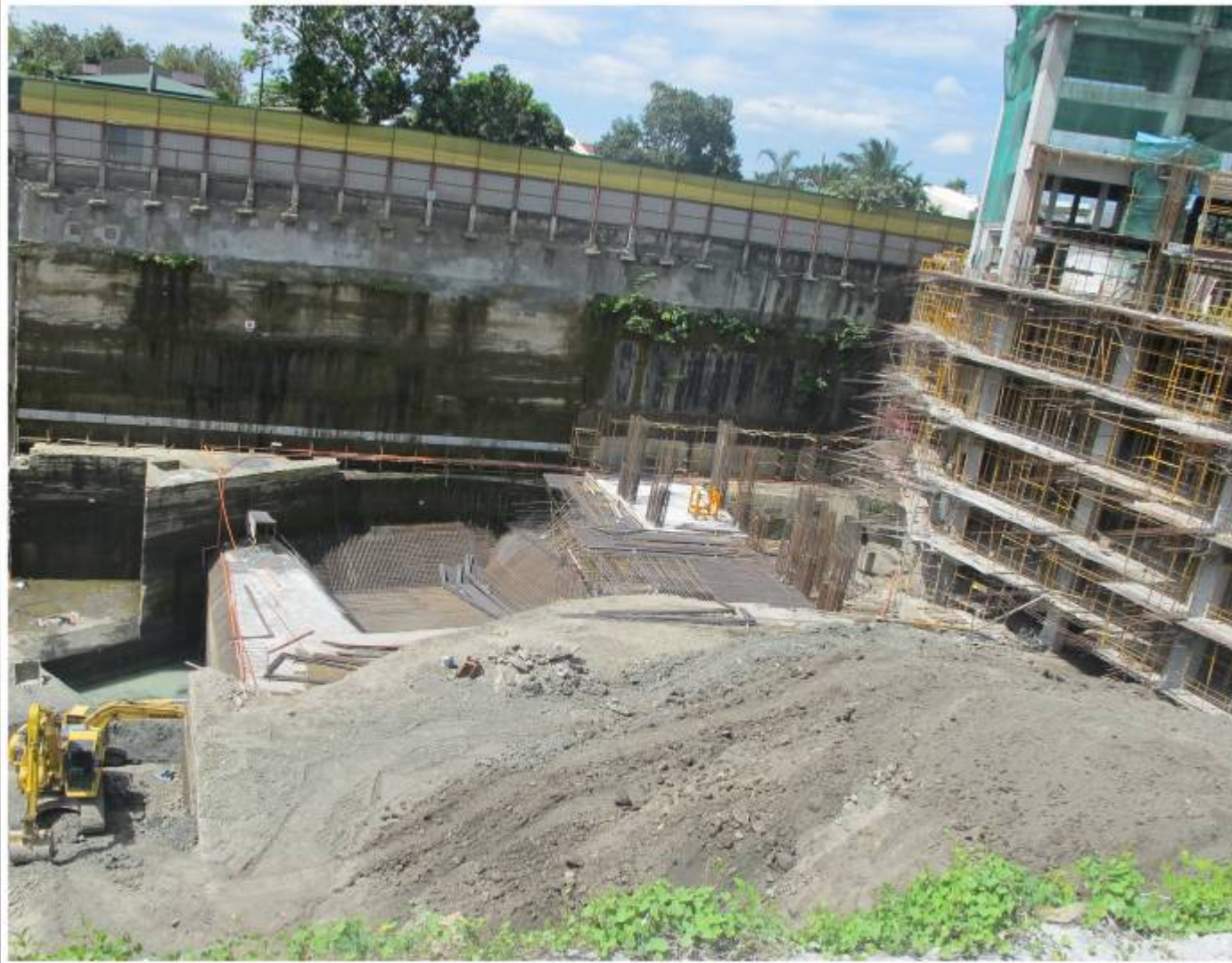
The Milano site with on-going rebar installation works
